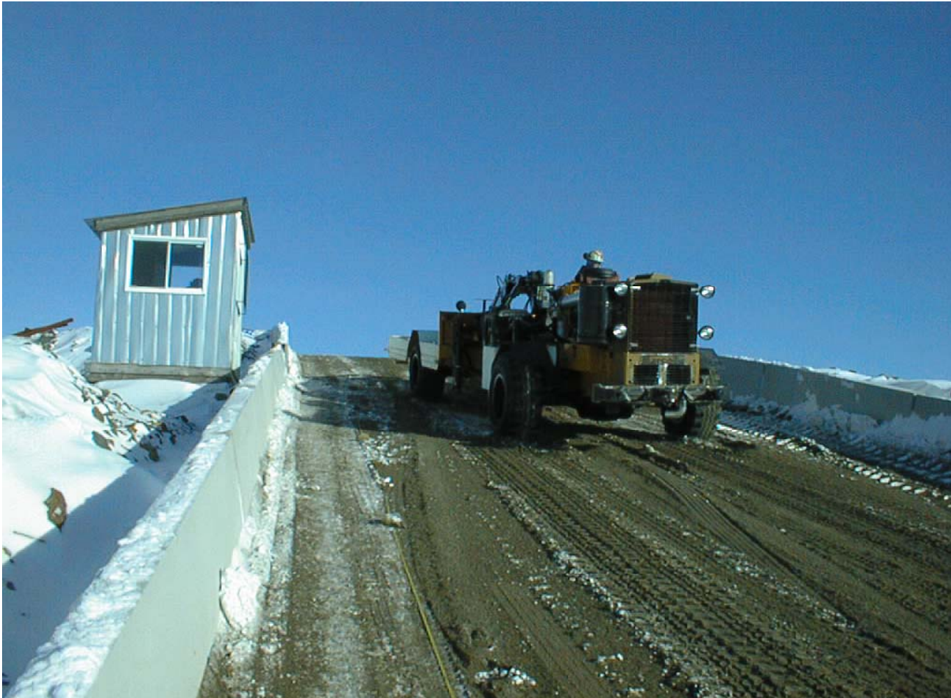
Copper Cliff Mine (North) 20% Grade Test Ramp
